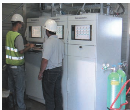
MIR FT mounted in air conditioned enclosure
