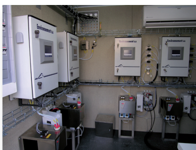
MIR 9000 - customized installation
